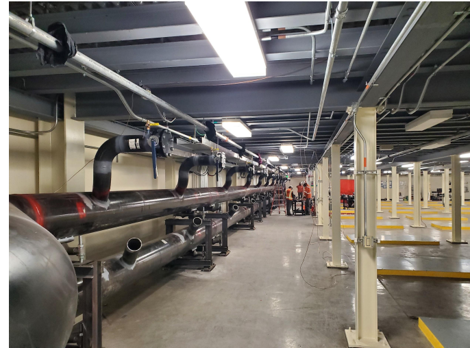
24" Mechanical Header Being Fitted & Welded
